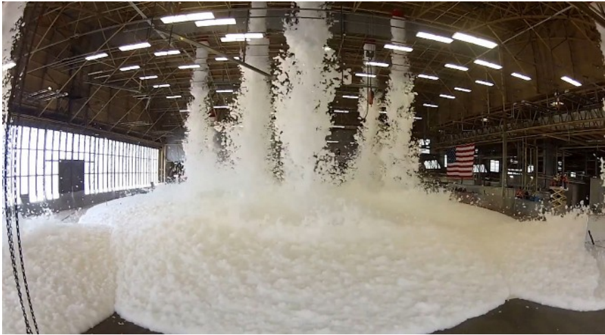
Figure 6: Flooding a hangar with extinguishing foam. 15 Original text: "PFAS appears in firefighting foam that has been routinely used on military bases nationwide" Photo: Department of Defense (DoD)
